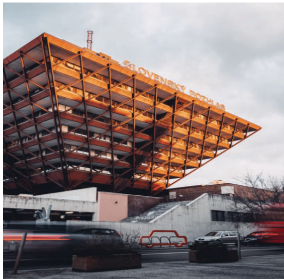
Building of Slovak radio
